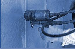
QUIK-SHIELD\* 112 XC is the preferred 2 lb. closed-cell, spray-applied, rigid polyurethane foam system on the market today. It is specially formulated for application to low temperature substrates, and is certified for use in the U.S. and Canada.
